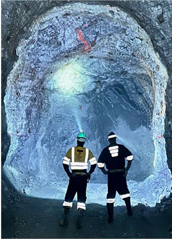
Ground Support Inspection
