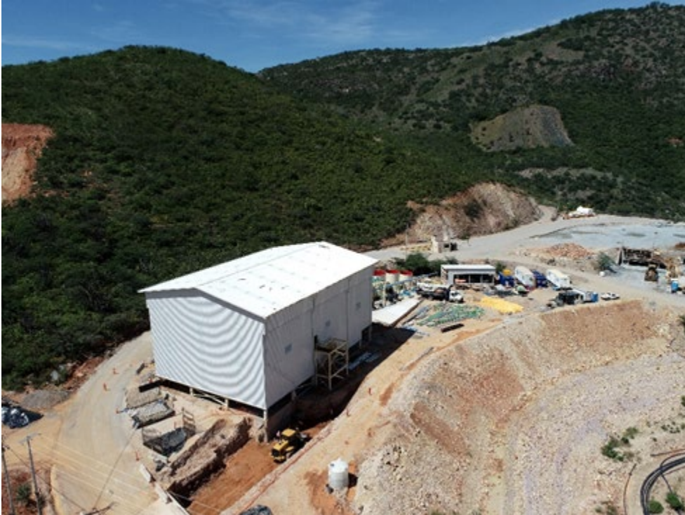
Figure 14-88: DDGM Tailings Filtration Plant.
