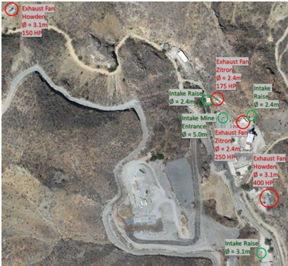
Figure 13-78: Ventilation Fans and Raise Bore Holes Installed at the Arista Underground Mine.
