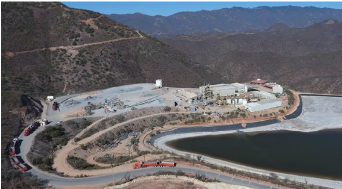
Figure 14-83: The DDGM Processing Facility.
