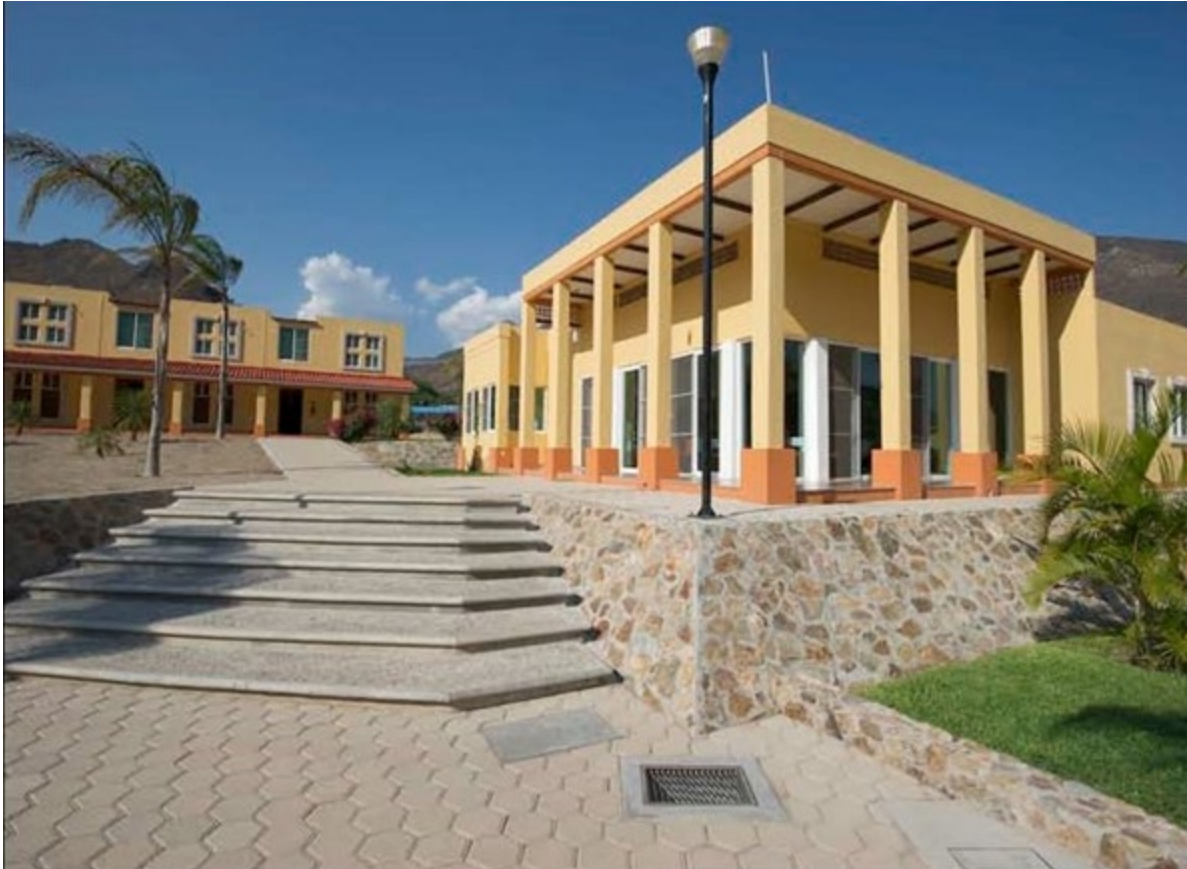
Figure 15-109: Recreation and Dining Hall Facility for Oaxaca Mining Unit (Tres Palmas) in the Town of San José de Gracia.
