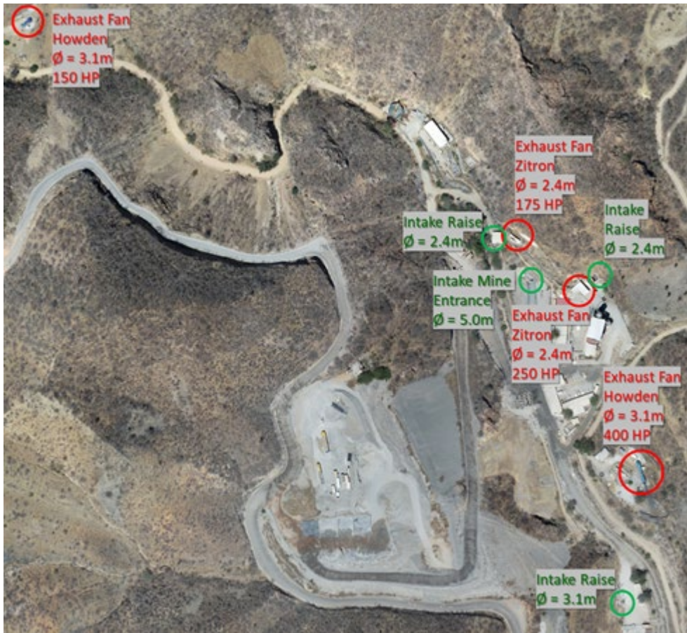
Figure 13.6 Ventilation Fans and Raise Bore Holes Installed at the Arista Underground Mine
