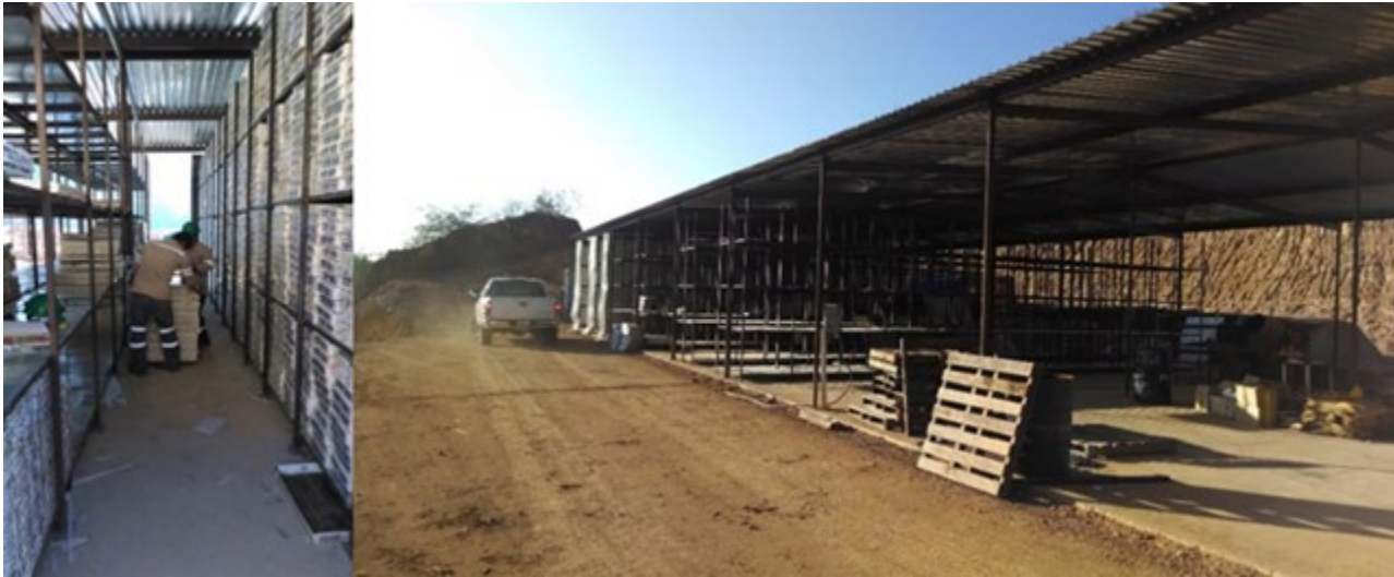
Figure 15.4 Core Storage Facility for the Don David Gold Mine Project
