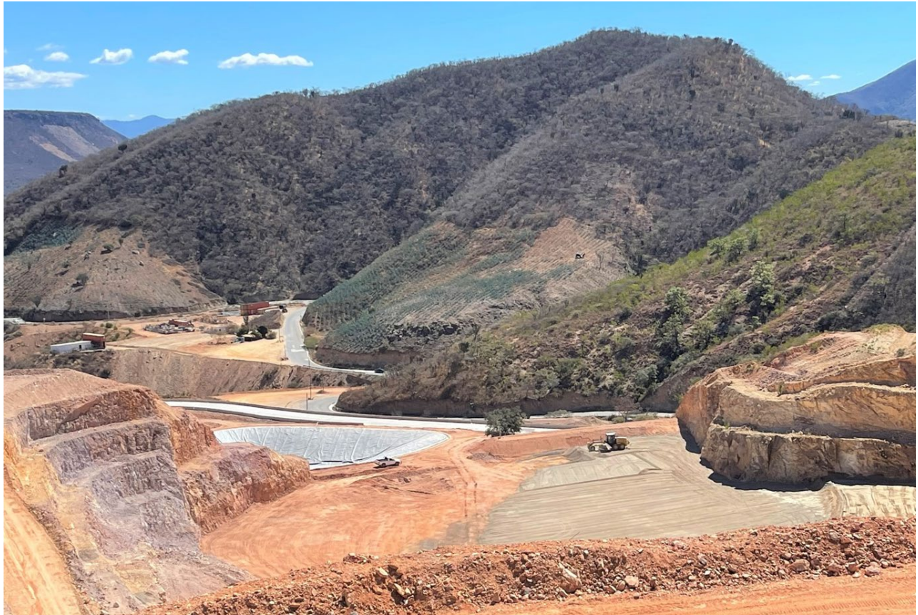
Open Pit and Dry Stack Facility
