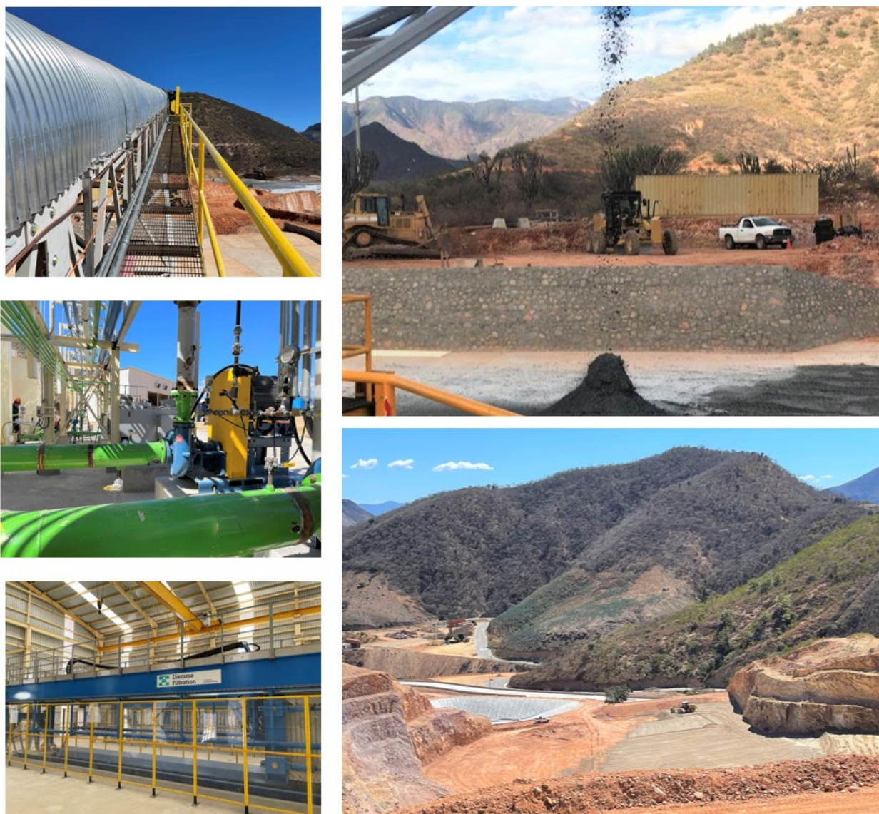
Dry Stack Tailings Filtration Plant and Dry Stack Area
