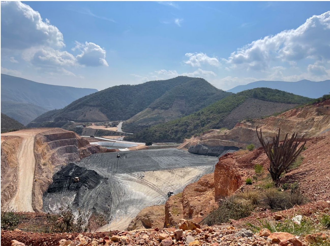
View of the Depleted Open Pit and Dry Stack Facility
